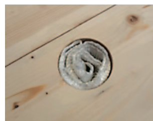
3. Transport situation with rolled-up loop in the blind hole
