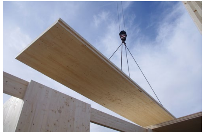
Lifting of KLH® TL panel
