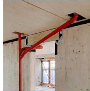
Figure 26. Shaft openings used for temporary drainage
