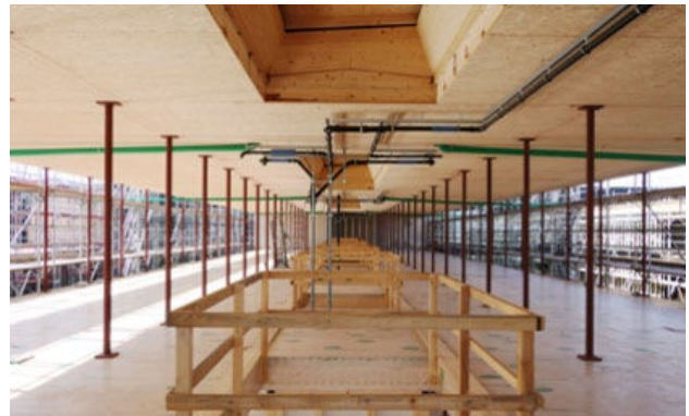
Figure 28. Secured and covered openings during construction
