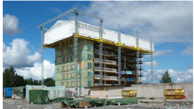
Figure 15. Temporary roof scaffolding, Berlin
