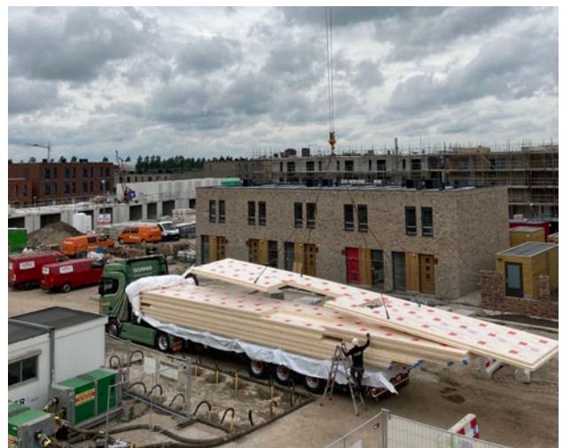
Figure 2. Floor panel lifting
