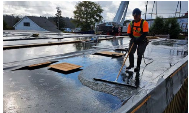
Figure 29. Removal of standing water from horizontal elements
