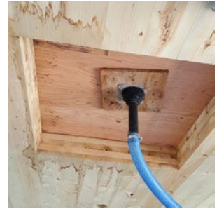
Figure 27. Temporary drainage for temporary drainage
