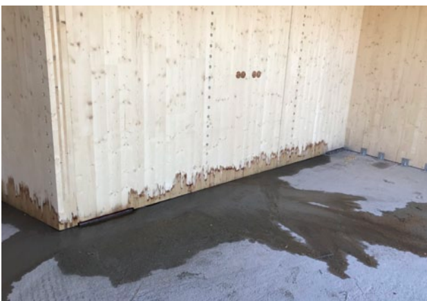
Rainwater absorption in unprotected end grain
