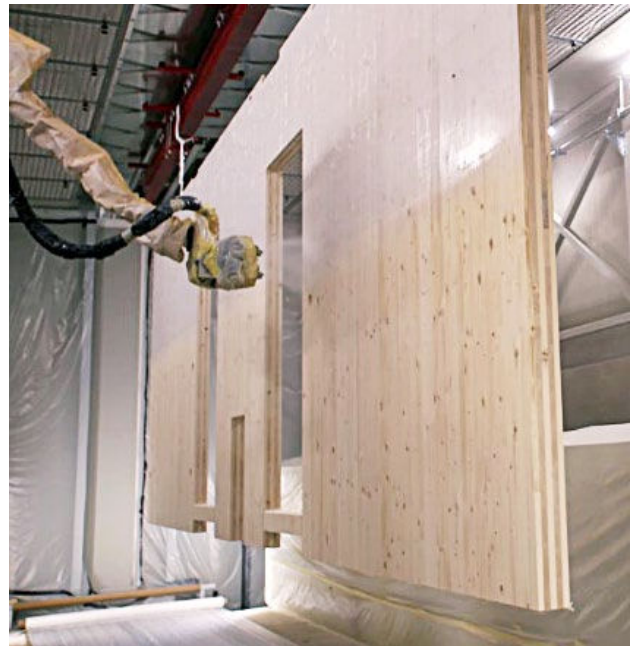
Application of white glazed surface
