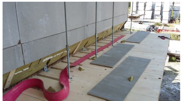
Wall-floor connection
