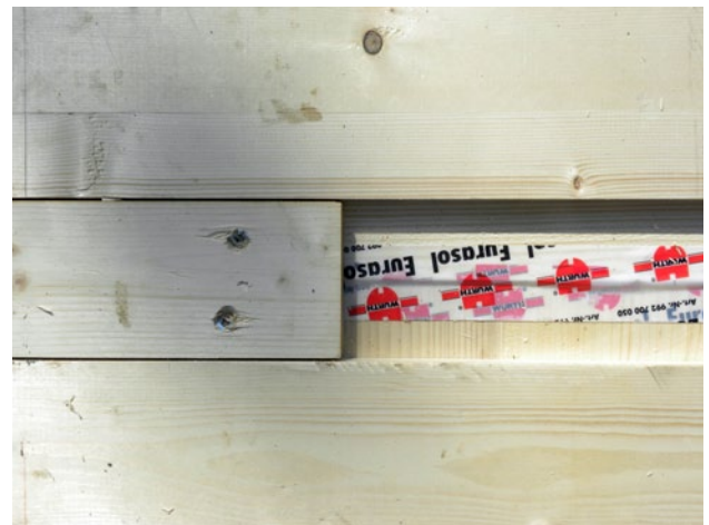
EXECUTION OF COVER BOARD
