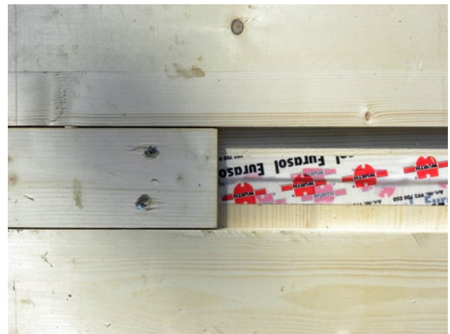
EXECUTION OF COVER BOARD
