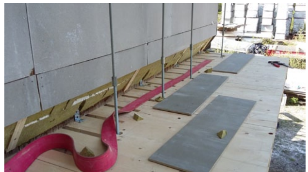
Wall-floor connection
