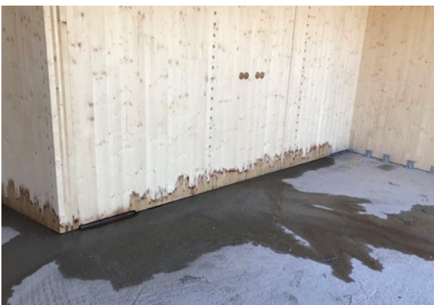
Rainwater absorption in unprotected end grain
