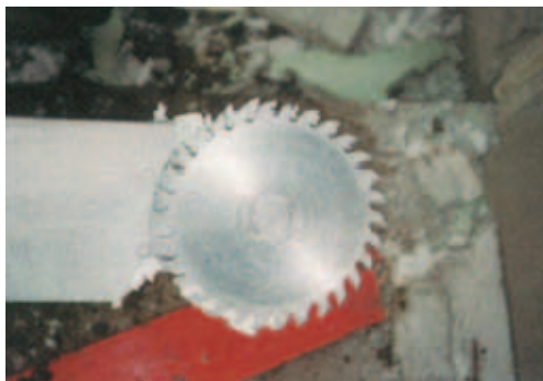
Fig. 18 – Repair work at a two-layer aerated concrete masonry wall with a double-sided saw blade on a 5 metre long blade [7.14]
